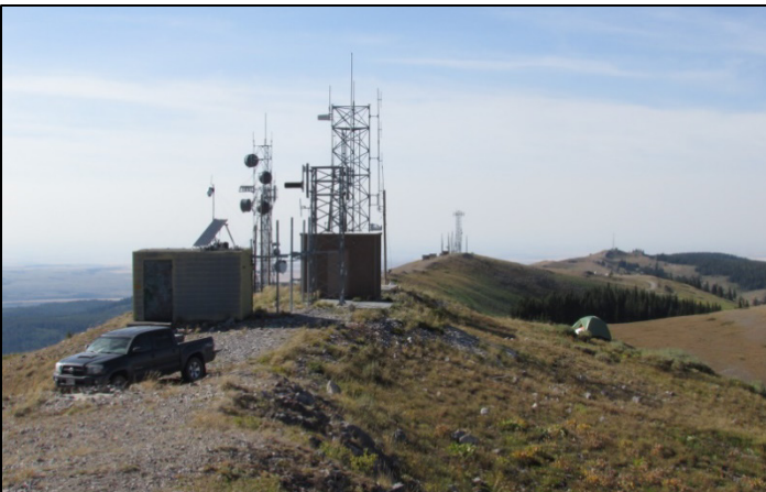
TOWERS STRETCH OVER A MILE ALONG THE TOP OF RELAY RIDGE IN IDAHO, WHERE I CHOSE TO WATCH THE 2017 TOTAL SOLAR ECLIPSE
