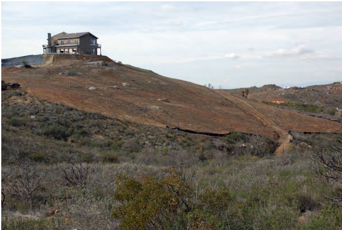
Figure 8. Three-hundred Feet of Clearance. Such bare ground can create a potential “bowling alley” effect, directing embers directly at the structure.
