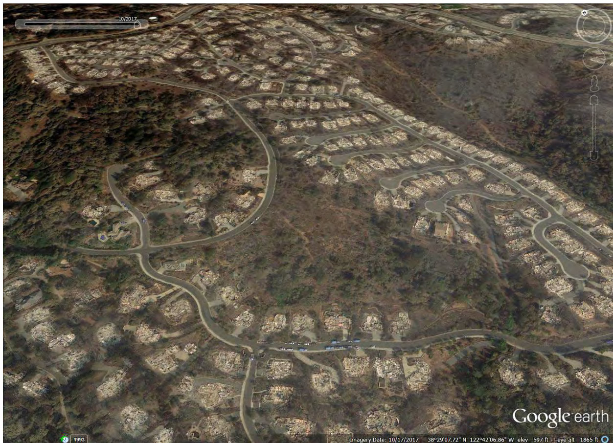
Figure 1. The devastation of the Fountaingrove II community in Santa Rosa during the 2017 Tubbs Fire was predictable. The city was warned this area was too dangerous to place homes. The area had burned in a wind-driven fire in 1964. In 2001, the city’s planning division issued a report concluding the development did not properly follow the city’s general plan’s goals and policies (Regalia et al. 2001).
