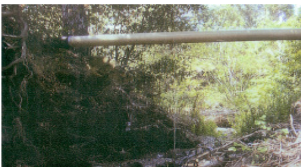
Look out below A replaced section of oil pipeline over Nipomo Creek.
