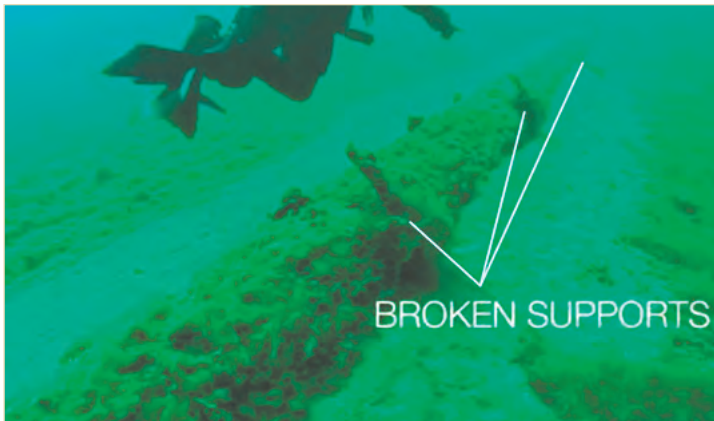
Diver checking out the condition of the ageing pipeline.
