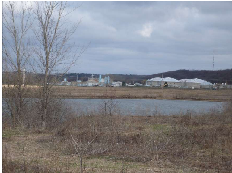
Cedar Rapids waste water treatment plant. Photo credit: Pam Mackey-Taylor
