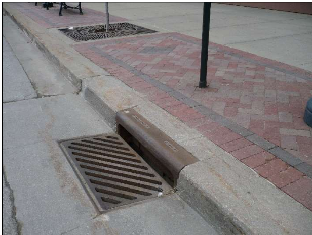
Storm sewer. Photo credit: Pam Mackey-Taylor
