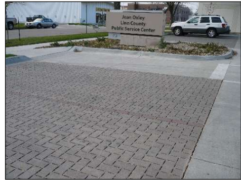
Permeable pavement, Cedar Rapids, Iowa. Photo credit: Pam Mackey-Taylor
