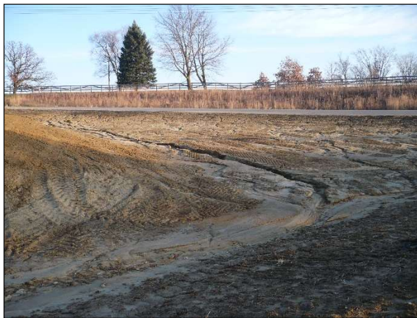
Storm water erosion on a construction site. Photo credit: Pam Mackey-Taylor
