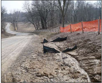
Silt fence at a construction site. Photo credit: Pam Mackey-Taylor
