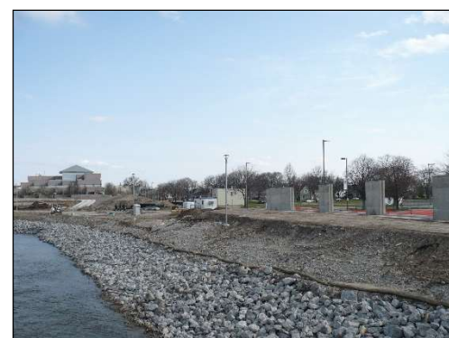
Riprap along the Cedar River in downtown Cedar Rapids, Iowa. Photo credit: Pam Mackey-Taylor
