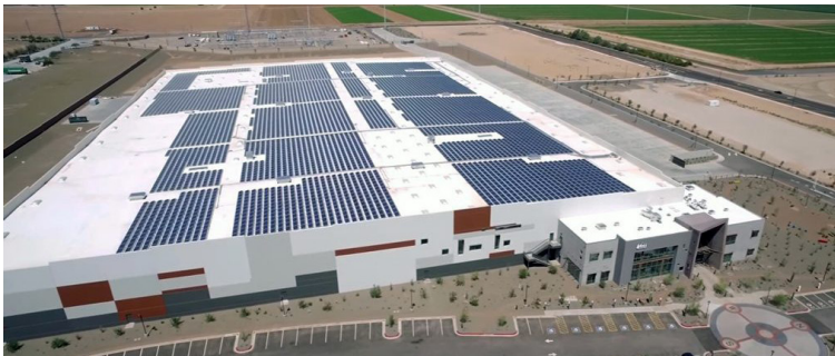
The REI Distribution Center in Goodyear features a 280,000-square-foot rooftop solar array. Learn more on page 2. Photo courtesy of REI Goodyear.
