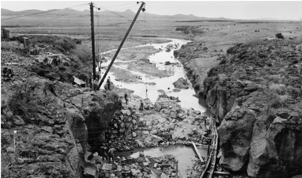
Figure 7. Construction of Sullivan Lake and Dam near Chino Valley (Call Number: dam132pq). Photo courtesy of Sharlot Hall Museum, Library and Archive, Prescott, Arizona
